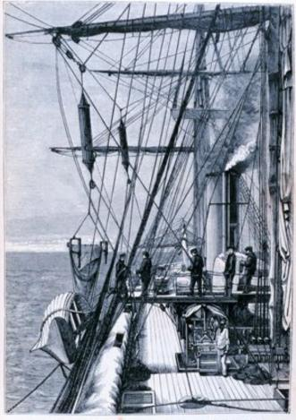
Fan 17 -- The Drolging and Sounding Arrangements on board the 'Challenger
